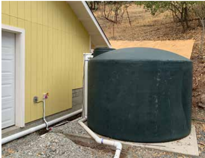
Example of a polyethylene or polypropylene (plastic) rainwater tank. They are the most common material used for residential rainwater systems and are available in various sizes.
