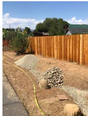
Photo 3: Gravel layers placed in trench.
