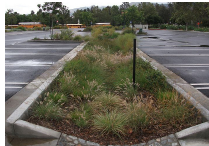
Fig. 15: Bioswale in Parking Lot Median Tool Type: Stormwater Reuse; Low Impact Development
