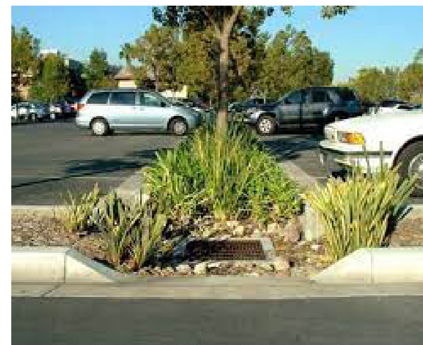
Image 2: Curb Cuts, an example of an LID project. (Source: State Water Board)
