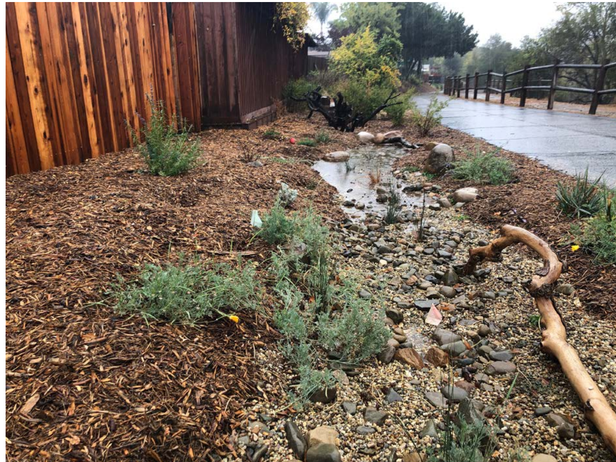
Figure 1: Land Resilience Partnership implemented bioswale. (Source: Watershed Progressive)
