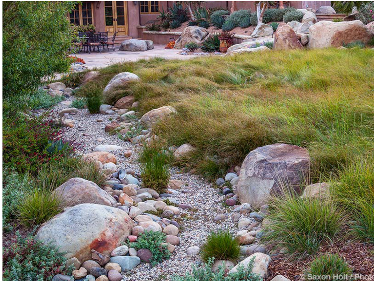
Image 1: Backyard bioswale, Carex lawn with dry creek rainwater bioswale for permeability (Source: photobotanic.com)
