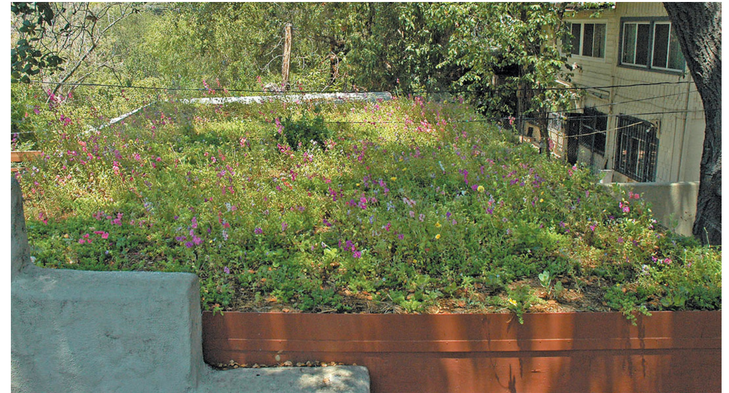
Image 2: Patio cover green roof with sedums and wildflowers in Altadena, California. (Source: Image by Bronwyn Miller; Design by Flower to the People, via Pacific Horticulture)
