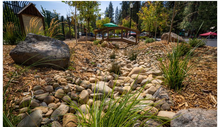
Photos: The bioswale captures the overflow stormwater, slows it, spreads it, then infiltrates it, replenishing groundwater supplies.
