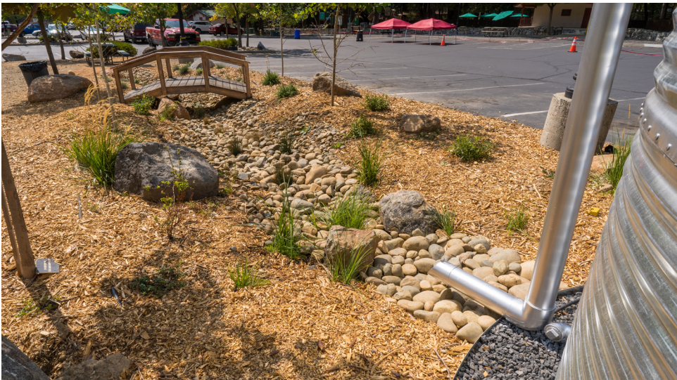
Photos: A rain tank collects rainwater and overflows to a bioswale.
