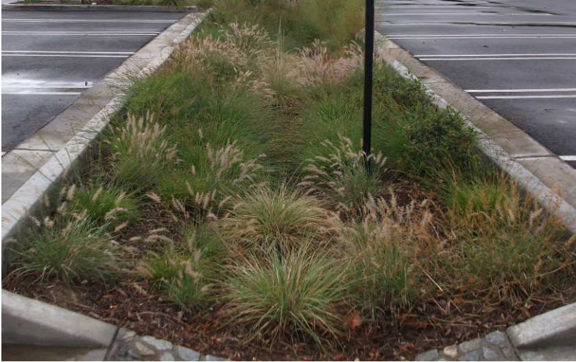
Photo: Typical bioswale in a parking lot. (Image source: greenportal.wca.ca.gov)
