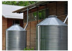
Dry conveyance system example Source: https://www.ul.com/services/certification-rainwater-catchment-systems-and-products
