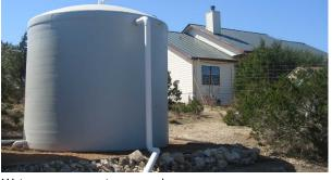
Wet conveyance system example Source: https://www.watercache.com/rainwater/residential
